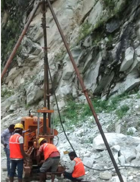
Fig. 2. Drilling in progress
