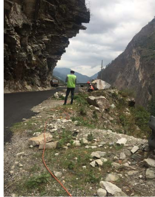
Fig. 3. Seismic Refraction test in progress
